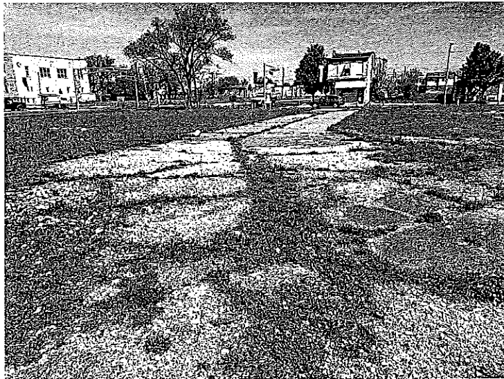
Image 6. Remnants of former industrial use.
