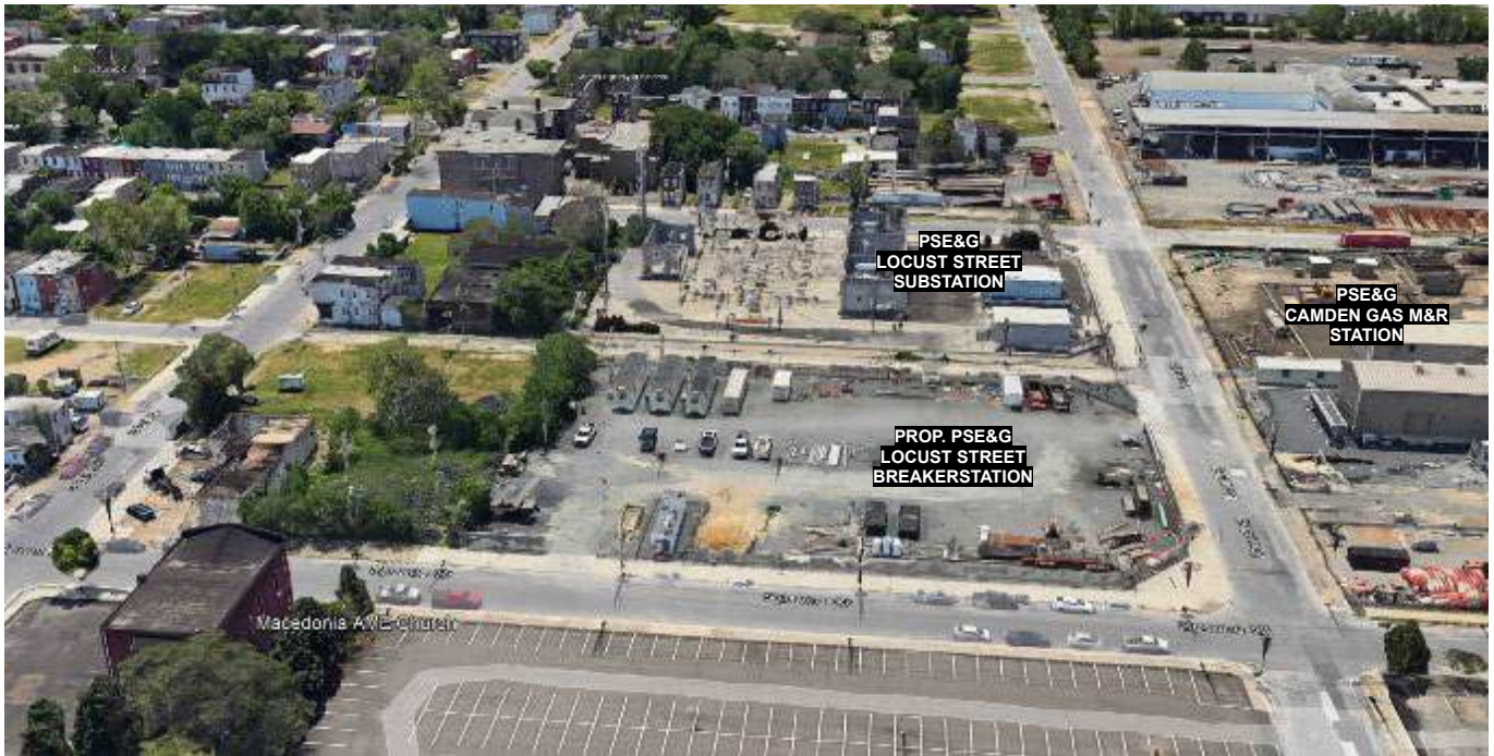
View #15 - Aerial View from Spruce Street looking south at Station
