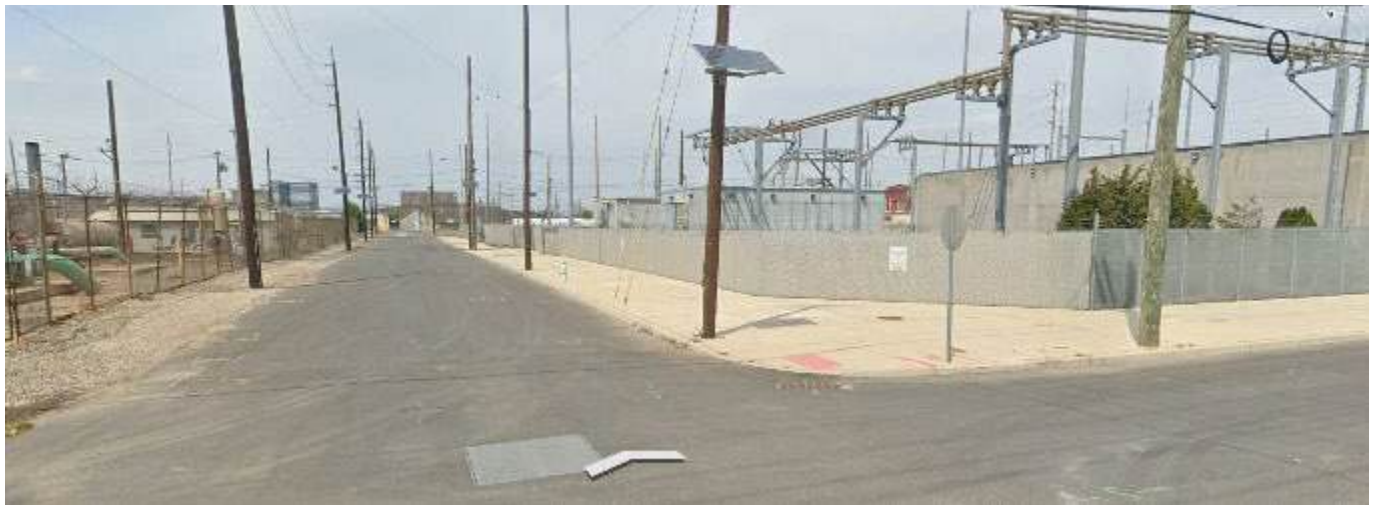
View #12 – View from intersection of Locust Street and Walnut Street looking northeast toward PSE&G Locust Street Substation on right
