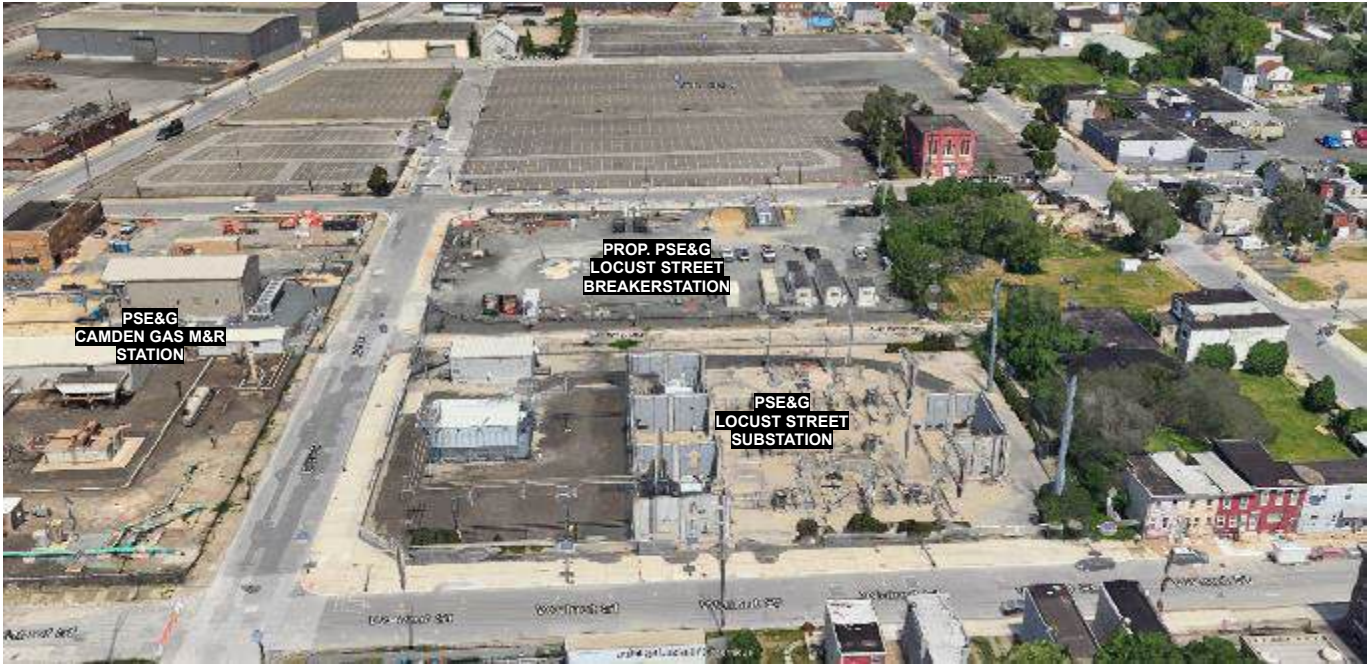
View #13 – Aerial View from Walnut Street looking north at Station
