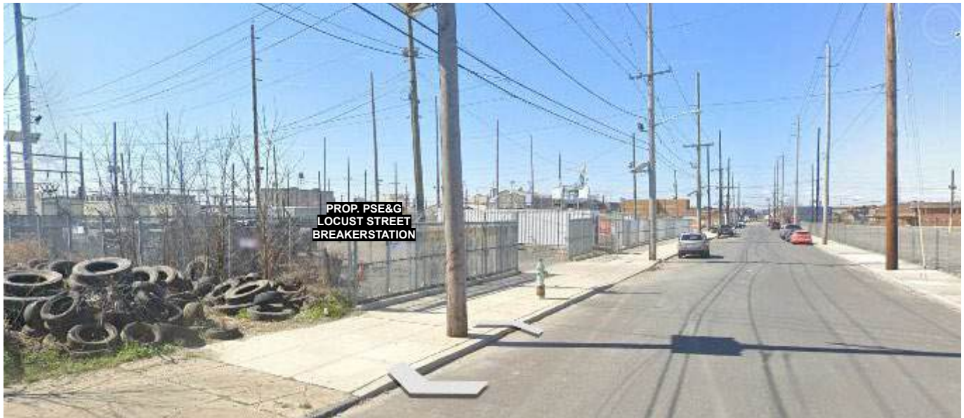
View #11 – View from Spruce Street looking southwest at Station on left
