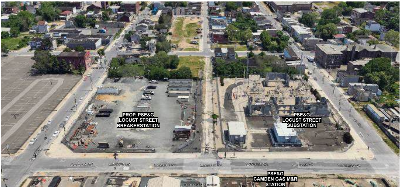
View #14 - Aerial View from Locust Street looking east at Station
