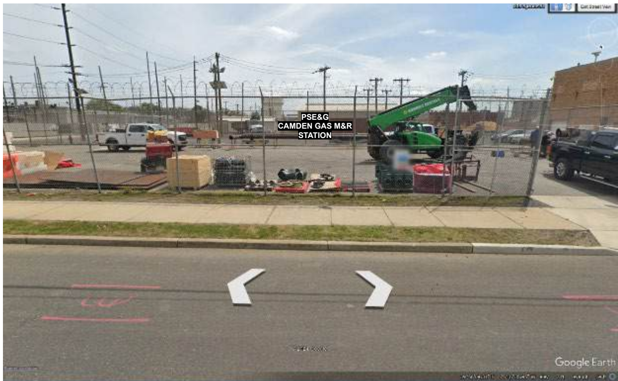
View #8 – View from 225 Spruce Street looking south at PSE&G Camden Gas M&R Station
