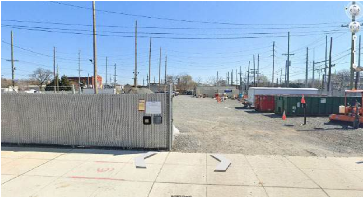
View #1 – View from Locust Street looking east into the Station property at the existing driveway
