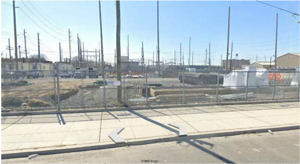
View #3 – View from Spruce Street, mid lot, looking south towards Station property
